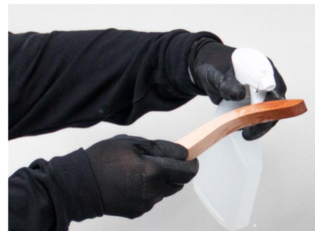
Use Finisher and a wooden spatula to tool the fresh joint. Only wet the spatula with Finisher. Do not spray directly onto the fresh sealant.
