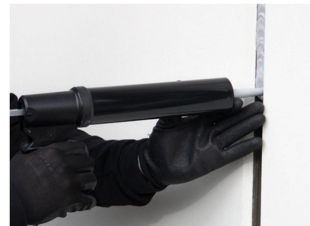
Apply the sealant at a steady pace and in sufficient volume to fill the joint. Make sure the sealant makes contact to both adhesion surfaces.
